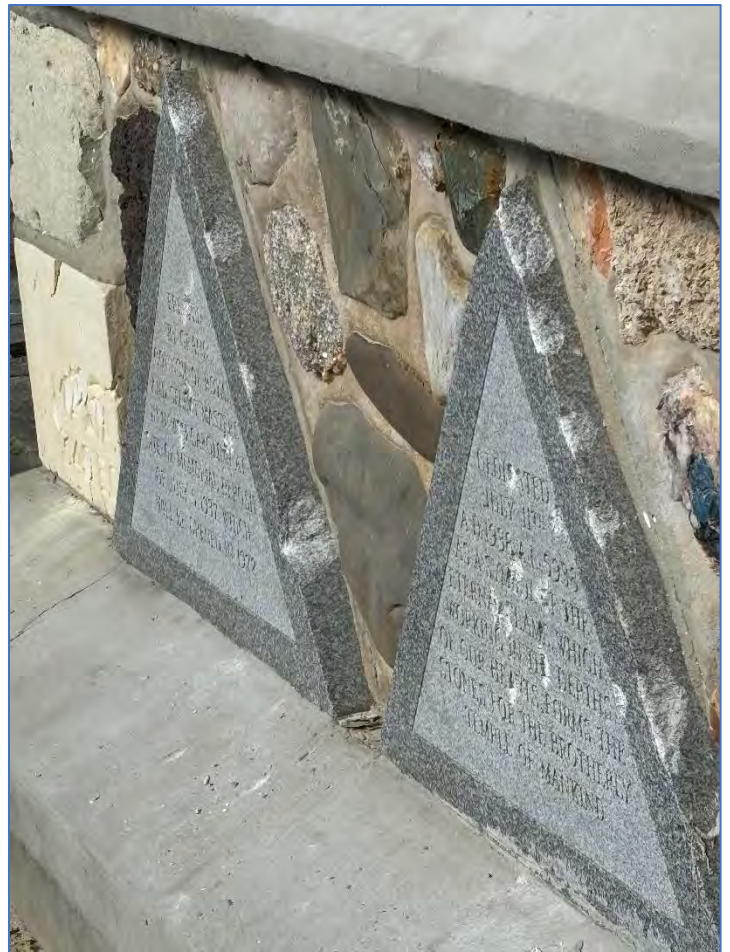
Damage was done to the stones on the marker inside the steel fence, which was forced open. Some of these stones are irreplaceable.
